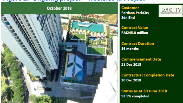
Figure 2: Ongoing project – Westside III Project
