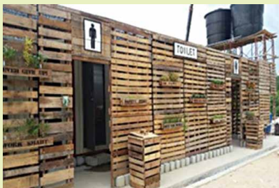
Used timber pallets as a wall divider
