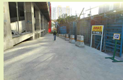
Concrete road barrier from concrete waste
