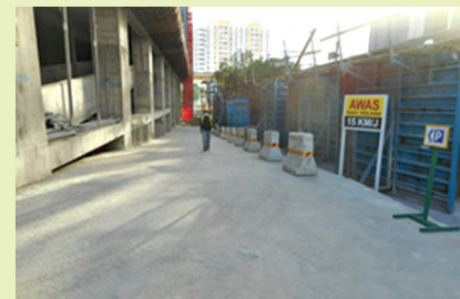
Concrete road barrier from concrete waste
