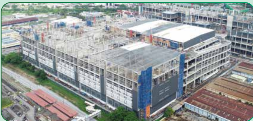
Logistics Hub – Plot B development under construction (approximately 73% completed), reflecting the Group's commitment to delivering high-quality and reliable built environments.
