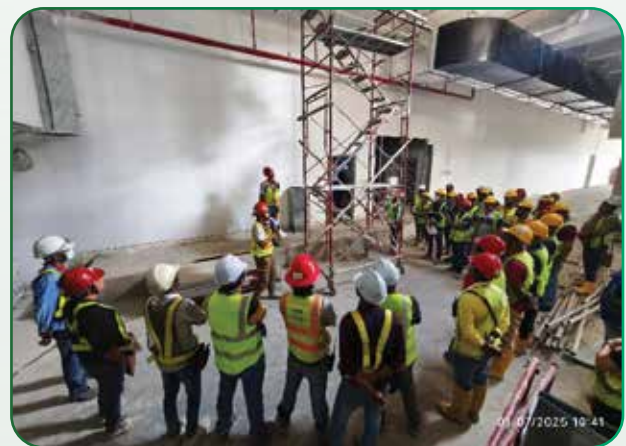
Workers undergoing scaffold safety training to reinforce safe work practices.
